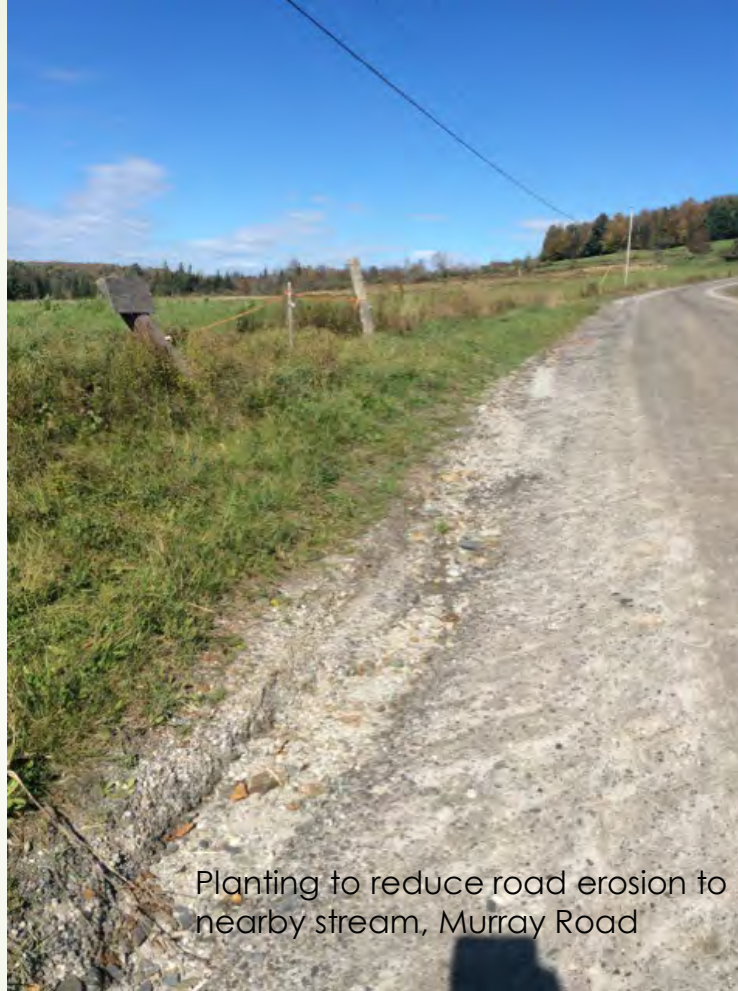
Planting to protect manage stormwater, Jacobs Road
