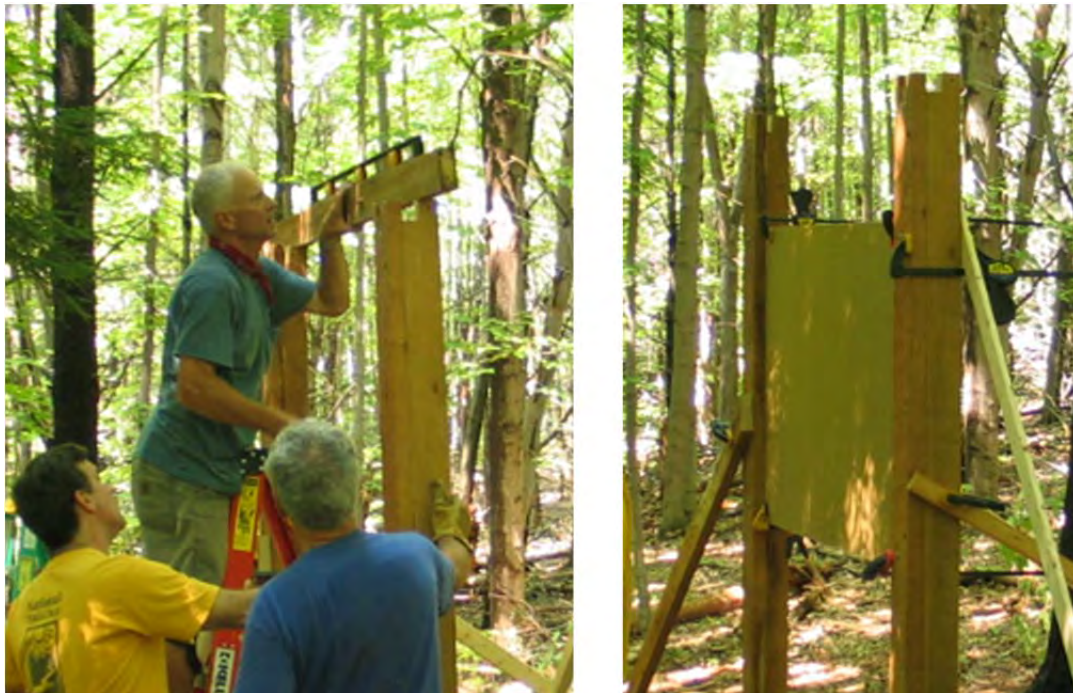
Figure 17. Aligning the tops of the legs (left) and squaring the legs using the MDO panel (right)
