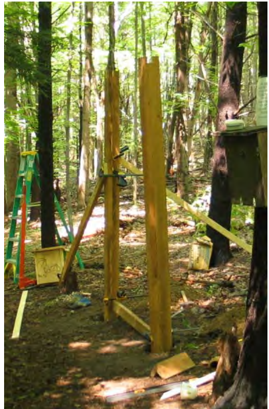
Figure 16. Aligning the legs
