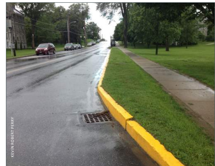
▲ Residential landscape strips and parking zones that are not heavily used can be retrofitted with larger rain gardens for stormwater management.
