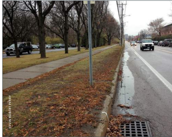
▲ Arterial roads with existing landscape strips can be redesigned to capture runoff.
