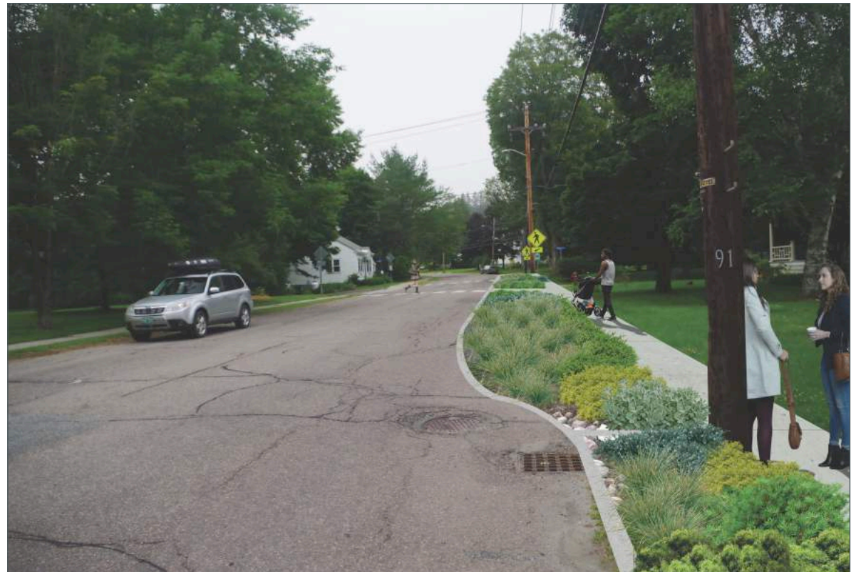
▲ RETROFIT OPPORTUNITY: The same residential street retrofitted with staggered mid-block stormwater curb extensions. Take note that the staggered condition helps create a traffic calming feature.
