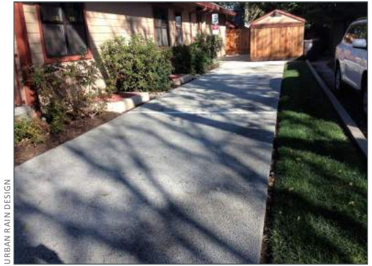
▲ EXAMPLE: A typical low-density residential driveway using pervious concrete.
