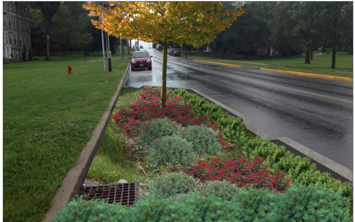
▲ RETROFIT OPPORTUNITY: The same residential street retrofitted with stormwater curb extensions, as well as additional street trees. In this example, the curb extension is only within the street leaving the existing curb in place.
