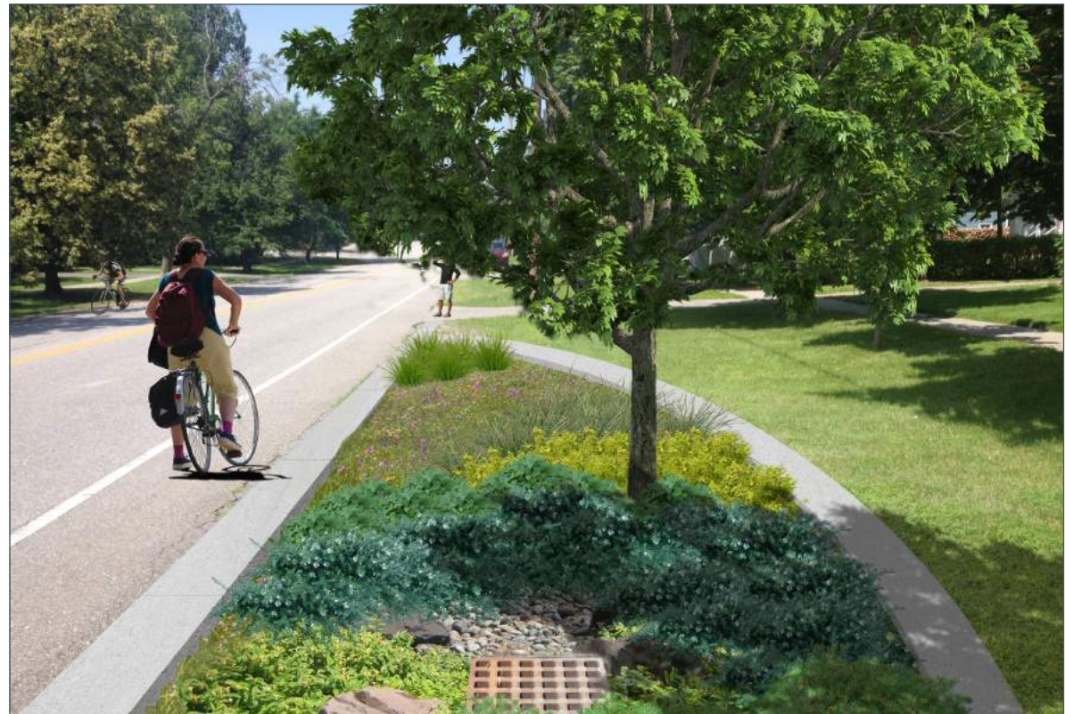
▲ RETROFIT OPPORTUNITY: The same residential street retrofitted with a rain garden. Take note that design incorporated an existing catch basin as part of the design.
