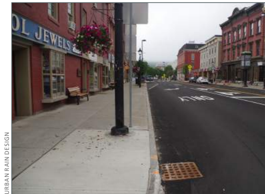
▲ EXISTING: A typical downtown main street with no on-street parking in Vermont.
