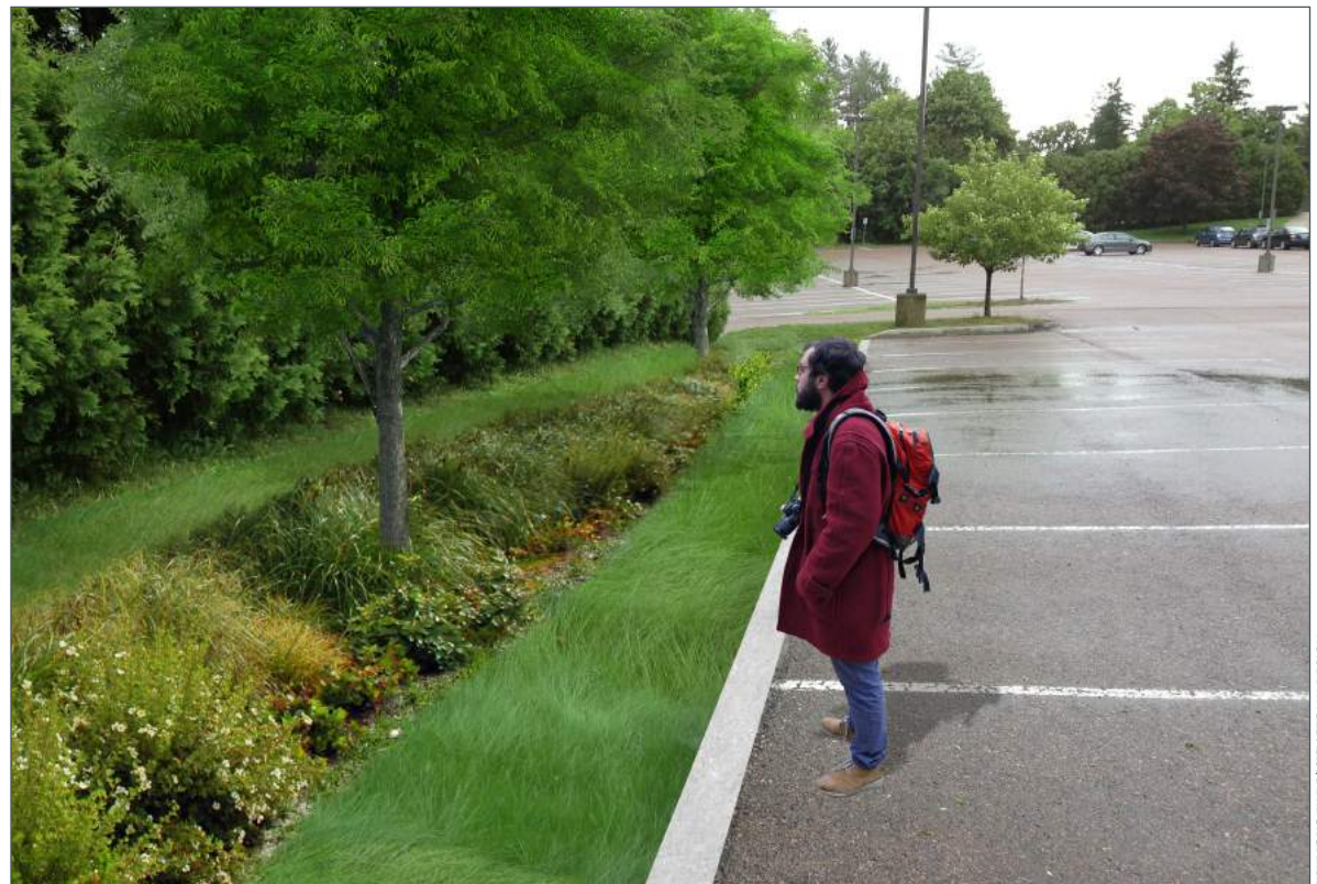
▲ RETROFIT OPPORTUNITY: The same parking lot perimeter space retrofitted with a vegetated swale. Notice the amount of plant diversity compared to just a mowed lawn space.
