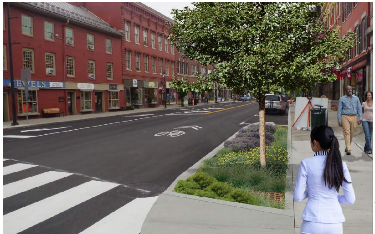
▲ RETROFIT OPPORTUNITY: The same downtown main street retrofitted with a stormwater curb extension.
